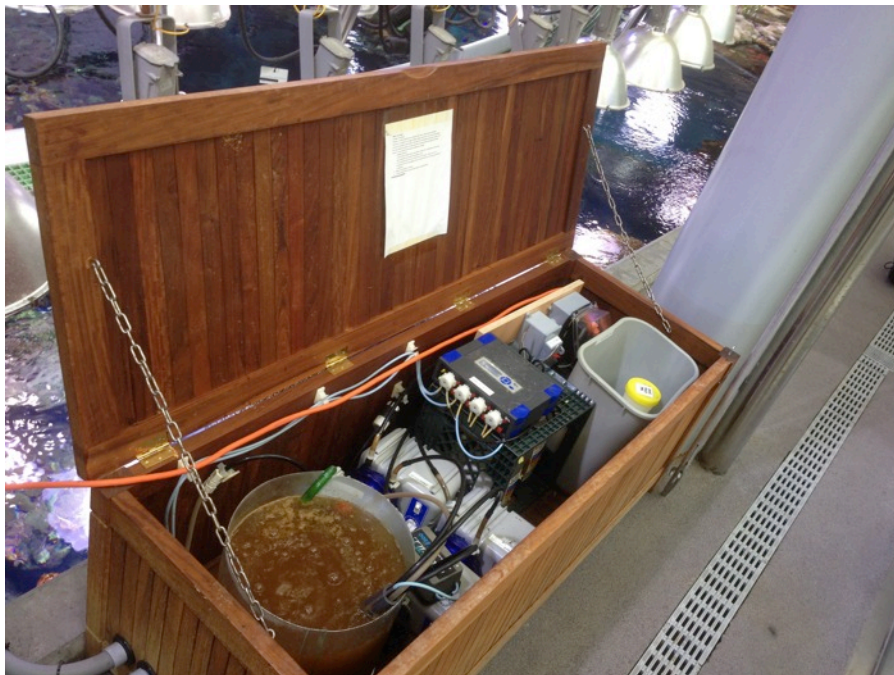
Photo 2: The chest above the exhibit holds the wet feed reservoir, the 4 peristaltic pumps, trace elements and doser, electrical switches and a container to hold foods that are fed during presentations. Photo R. Ross
